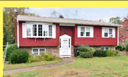
SWANSEA Raised Ranch $329.900
